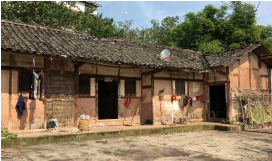
Before the 1990s, most houses in rural China were built with rammed earth and wood.
