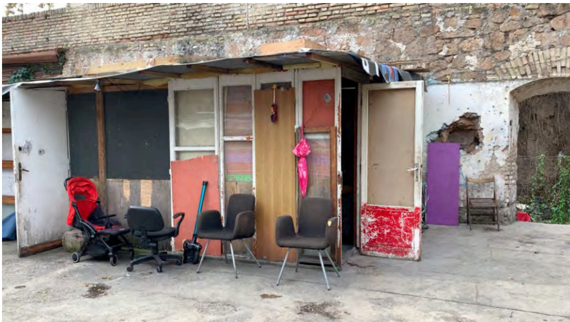
At the former Mira Lanza factory, doors and windows used as walls to allow more light into the dwellings.
