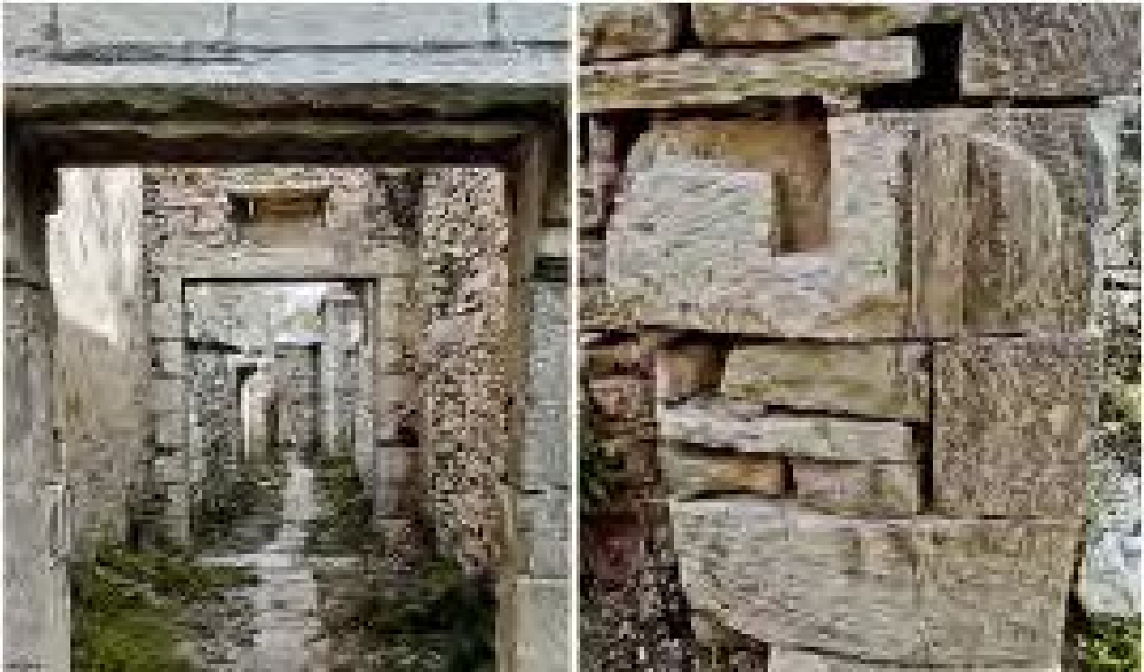
A rural house in Fangyu village, approximately built in 1890. Its stone awaiting salvage.
