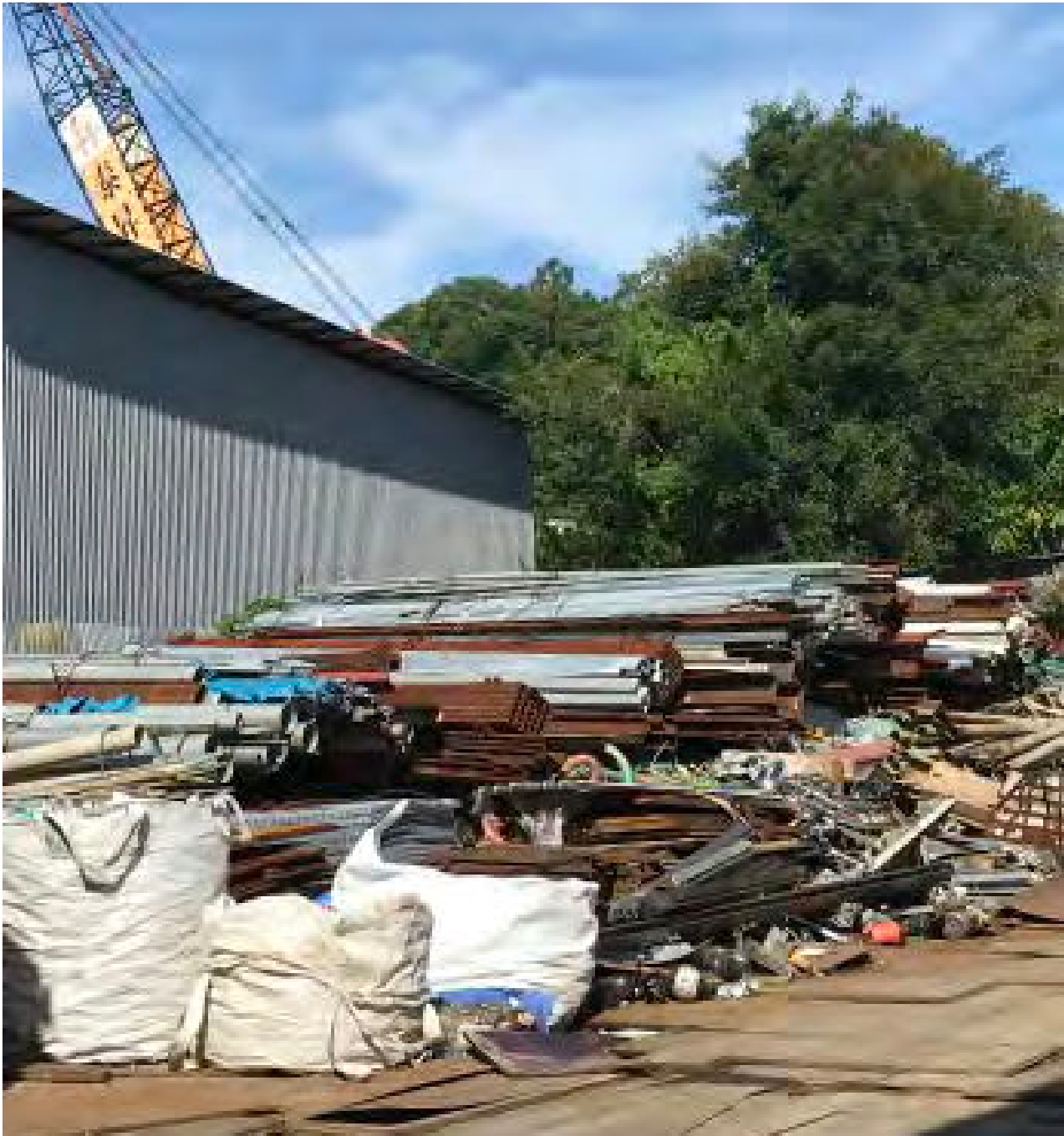
An accumulation of reusable metals, including I-beams and pipes, are piled up right next to the entrance.
