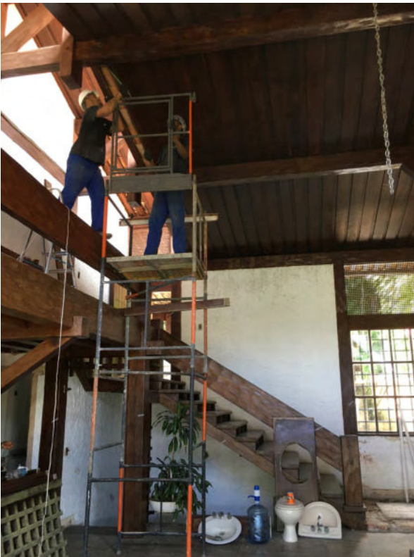
Arquivo workers dismantling wooden ceiling panels.
