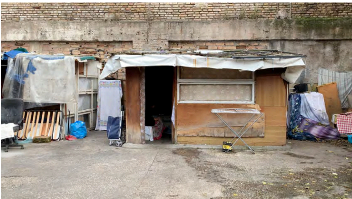
Euro-pallets used as weight to hold the tarp on top of the structure, placed directly above the insulation foam.
