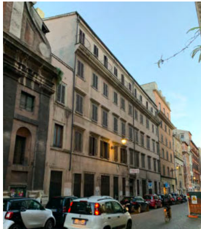
Abandoned public building belonging to the Statal Aministrative office. Apartments used to be rented out to the office workers.
