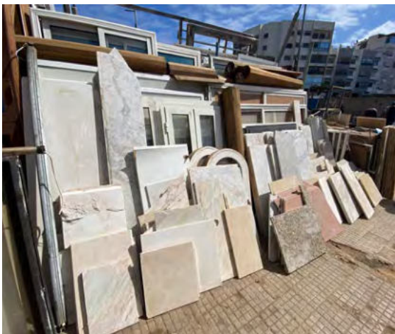
Materials exposed in the street and left at night.
