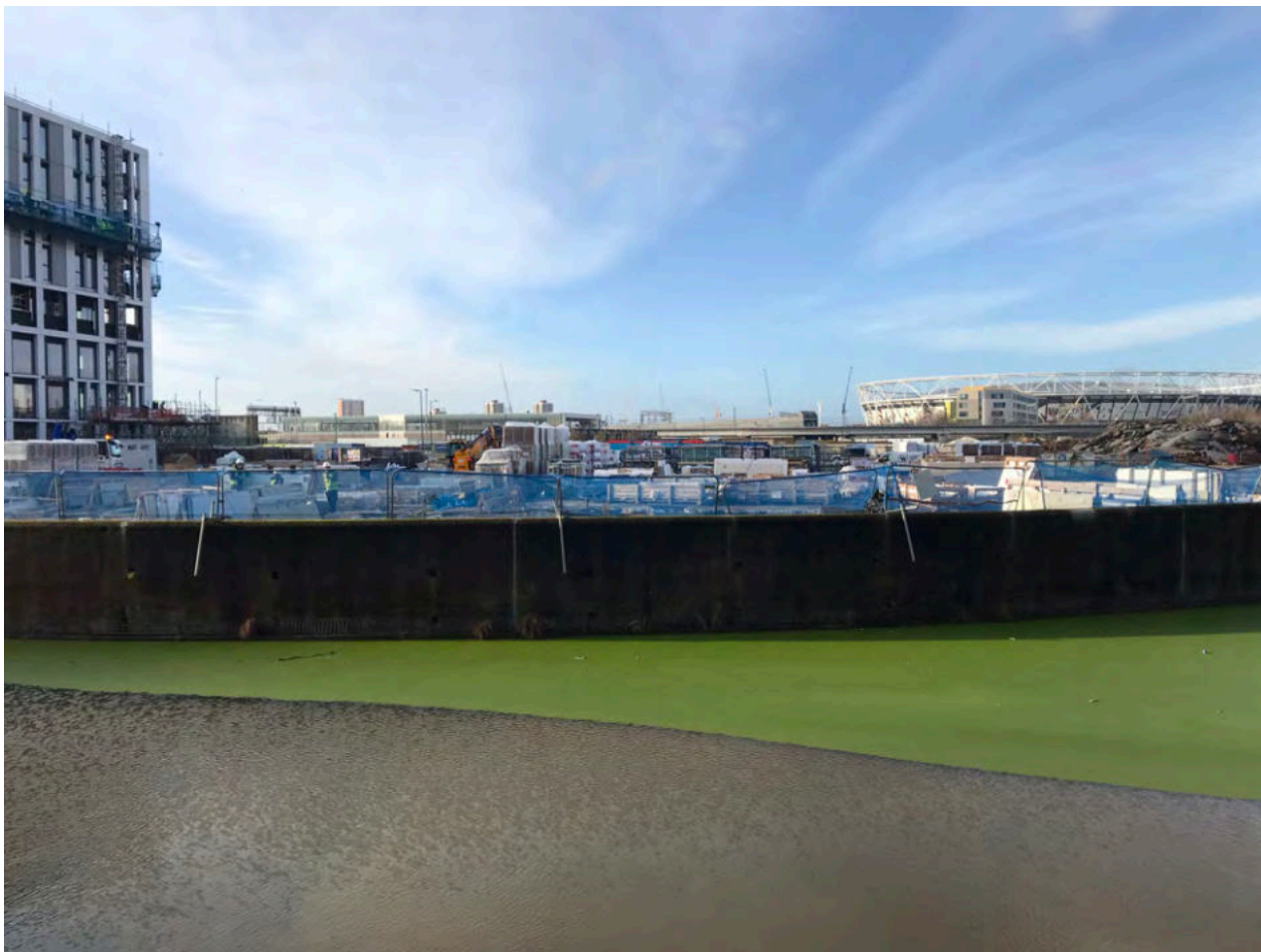
London E15: Development with opening to the Bow Back River canals, with potential to use the waterways for material transport and waste disposal.
