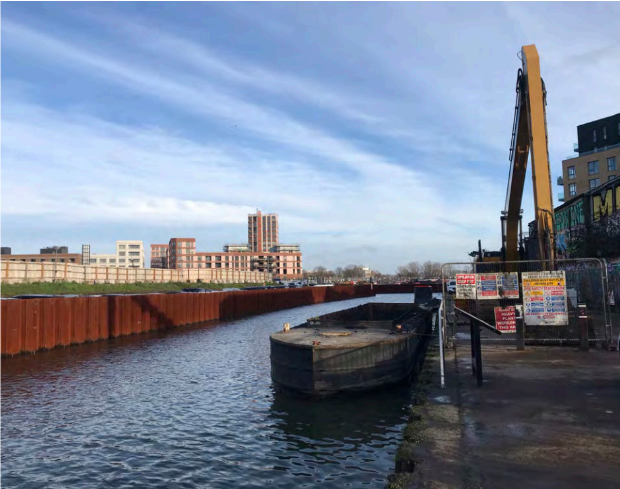
Water and dock construction site, cranes loading dumb barges with waste materials.
