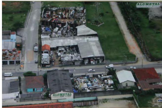
Sparked by a reclamation yard in the city of Curitiba, Alumental is the largest material reseller in Florianopolis and have been operating since 1999. Although Alumental has brought more awareness to the re-usability of materials, it is still one of four material reuse yards in Florianopolis.
