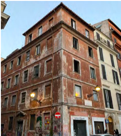
Roma Capitale's administrative service building. Structure made out of brick with plaster rendered walls and wooden doors and windows and roof of U-shaped tiles .
